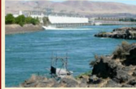
1952 The Dalles Dam construction begins
